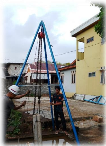
a. Install small-pile cluster
