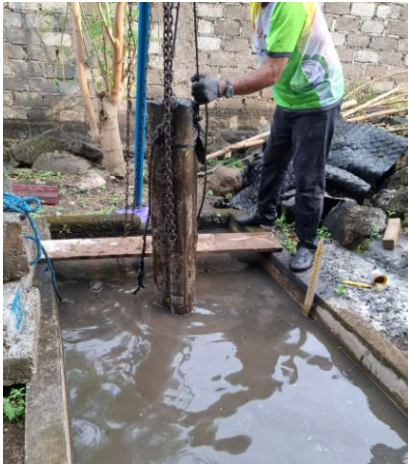
c. Remove small- pile cluster
