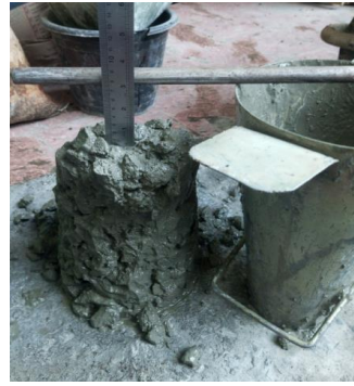
b. Check concrete consistency
