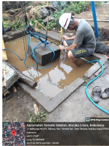
b. Observe deformation due to loads
