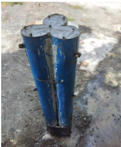
a. Fabrication process of small-pile
