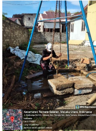
d. Removed the concrete blocks
