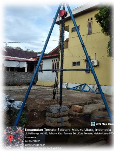
c. Complete step of static loading with concrete
