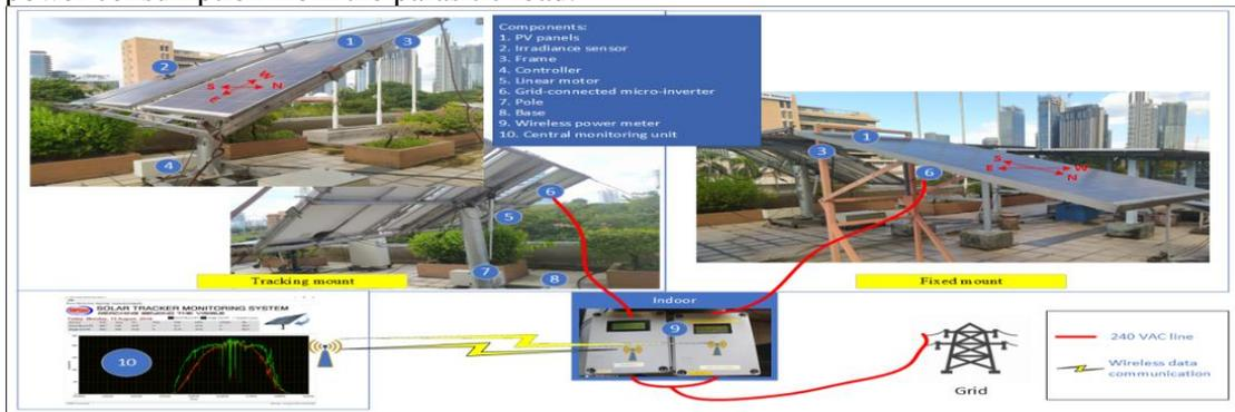
Fig. 2. Single-axis tracking system and fixed mounted PV components
